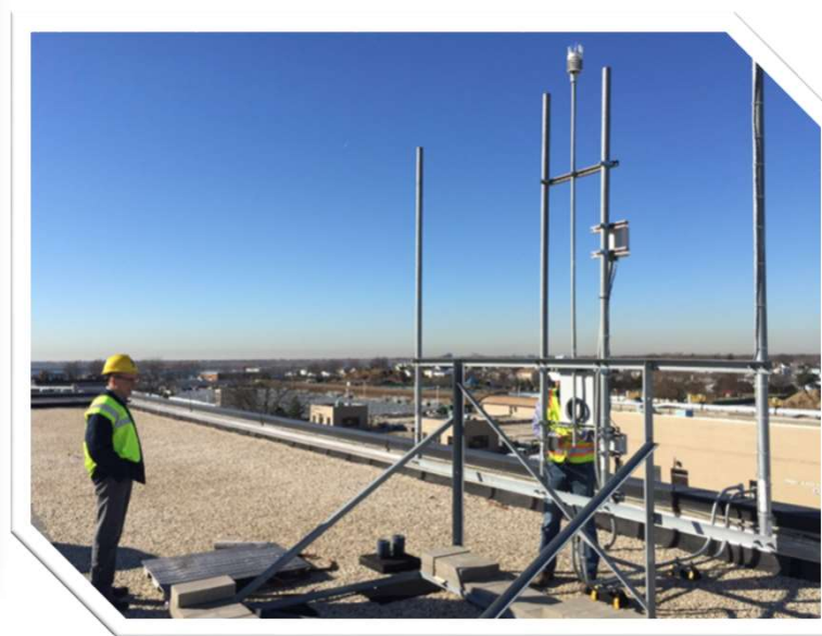
Central Radio Antenna & Weather Station
