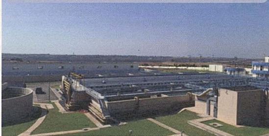
Station de traitement Oum Azza (5 m 3 /s)
